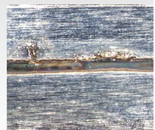
Material defect detected by SWM-2.
